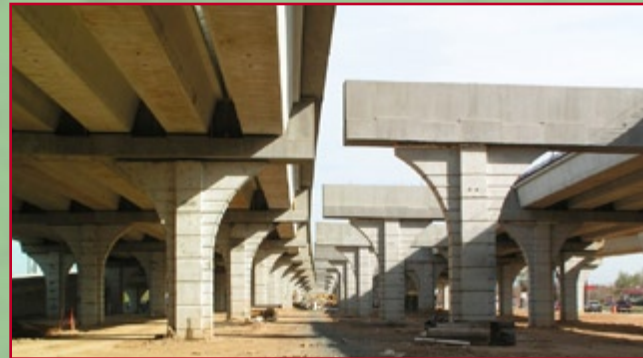
Contract A - Columns for the new IH 10 eastbound mainlanes bridge over Katy-Fort Bend and US 90 (looking east).
