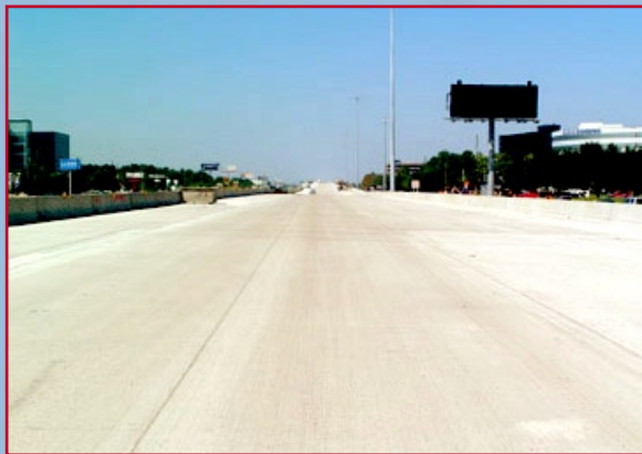
▲ Recently completed IH 10 westbound mainlanes east of Park Ten (looking west)
