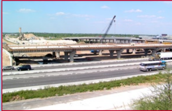
▲ An aerial view of the IH 10 westbound mainlane bridge at SH 99.
