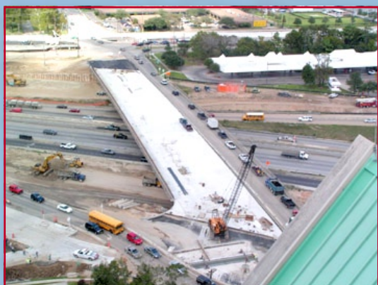
▲ Aerial view of construction of the new North Post Oak bridge.
