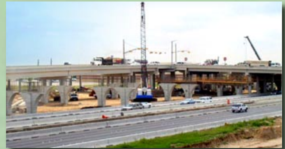
Overview of IH 10 construction at SH 99
