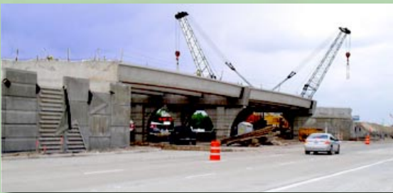
Construction of Park Ten Boulevard intersection
