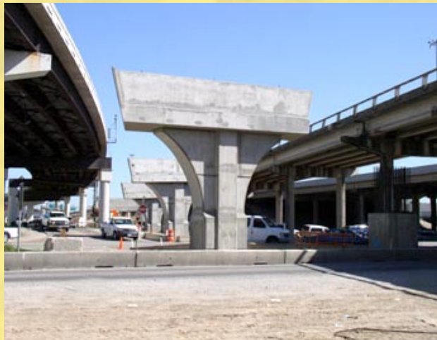
Columns for IH 610 to IH 10 westbound direct connectors
