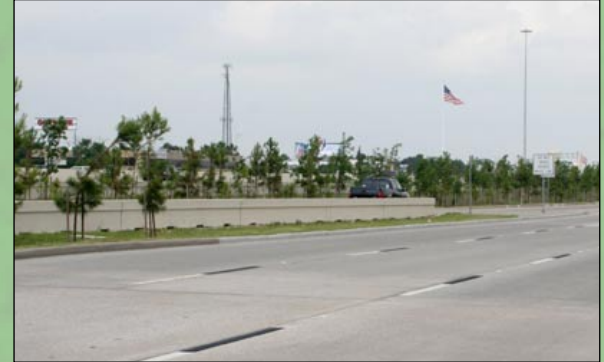
Contracts A and B - The completed landscaping along the IH 10 westbound frontage road west of Fry Road
