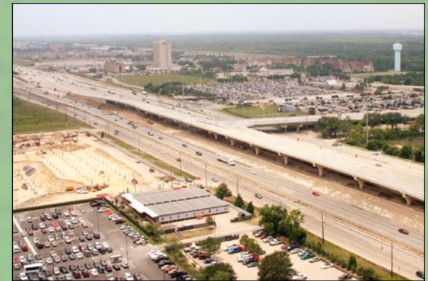
Contract C1 - The new IH 10 mainlanes bridge ramp to and from the Addicks Park and Ride
