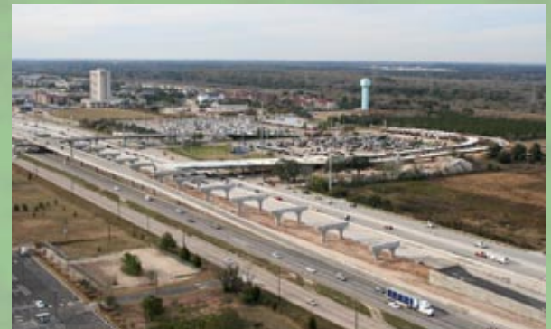
Contract C1 - Aerial view, looking west, of the new IH 10 mainlanes T-ramp to/from the SH 6/Addicks Park & Ride under construction
