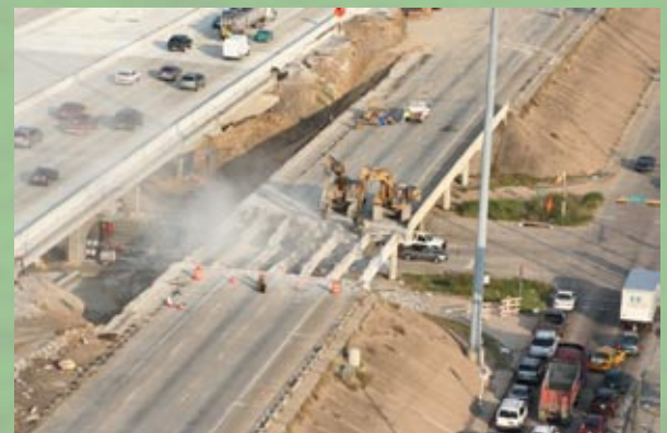
Contract C2 - The existing IH 10 eastbound mainlanes bridge over Kirkwood being demolished
