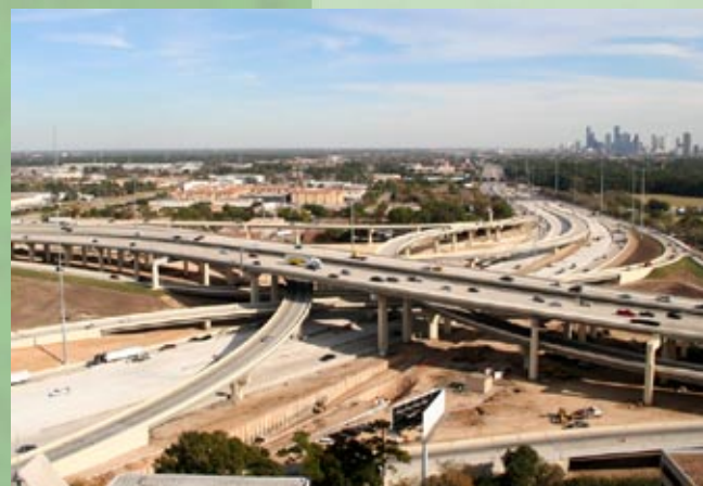
Contract F - Aerial view, looking east, of the IH 10/IH 610 interchange
