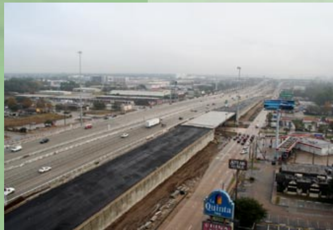
Contract D - Aerial view, looking east, of the new IH 10 eastbound mainlanes bridge over Wilcrest
