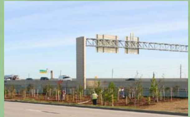
Contracts A & B - Contractors planting trees in the vicinity of the intersection of IH 10 and Barker Cypress.
