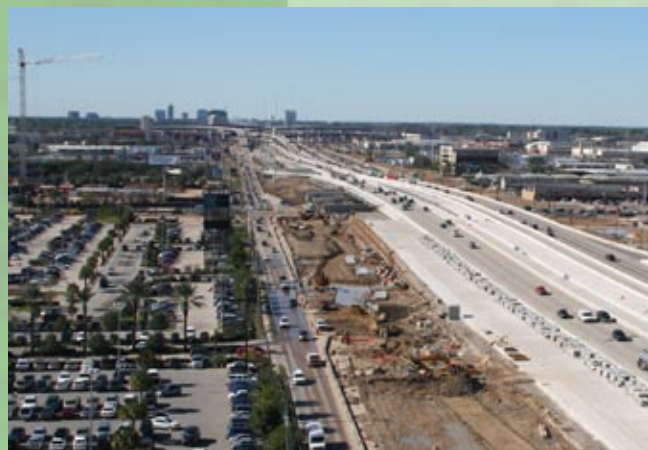
Contract E1 & E2 - Overview, looking west, of the construction area showing IH 10 eastbound and westbound mainlane traffic on new pavement near Gessner
