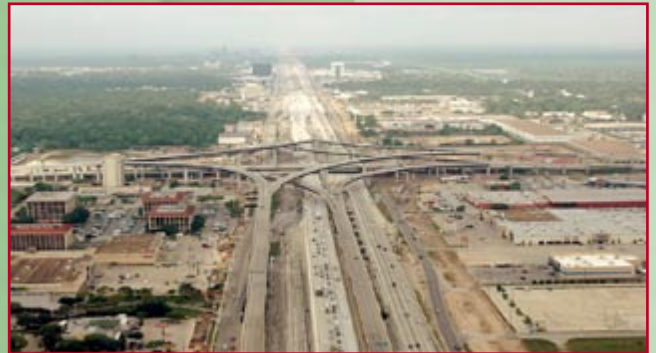
Contract D - Aerial view, looking west, of the IH 10/Beltway 8 interchange.
