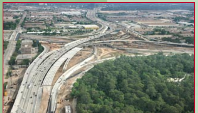
Contract F - Aerial view, looking north, of the IH 610 mainlanes bridge over IH 10.
