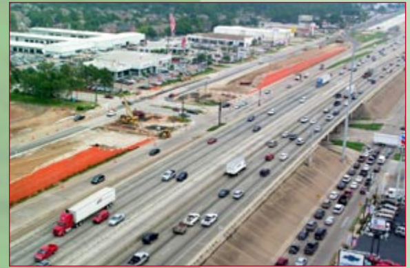
Contract C2—Overview of construction at IH-10/Kirkwood
