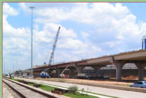
Contract A—New IH-10 westbound mainlanes west Katy Fort-Bend
