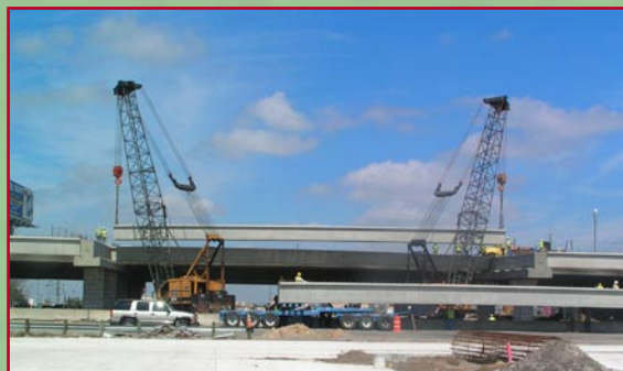
Placing beams for the IH 10 mainlanes at Fry road
