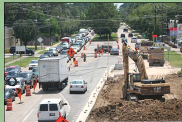
Contract C2 - Crews excavate and grade the southbound lanes of Kirkwood (looking south).
