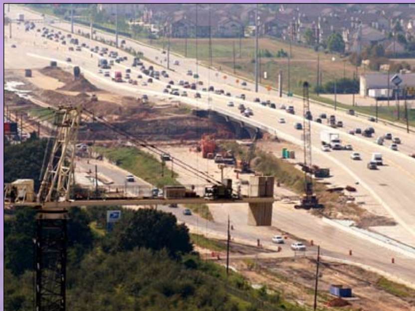
Aerial overview of construction at IH 10 and SH 6 highlighting the recent demolition of the old IH 10 eastbound mainline bridge over SH 6 in preparation for the construction of the new structure.
