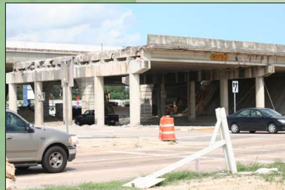
Contracts E1 and E2 - As part of the intersection replacement occurring within these contract limits, the bridge structure over Antoine is being demolished.
